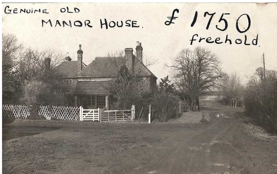
The Old Manor House, junction of the Drive and the Drove
